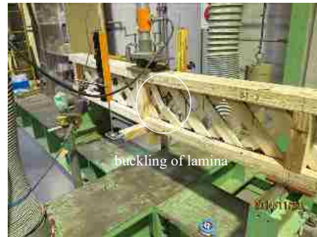
Fig. 3-14 Situation after loading
