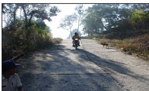
Fig.40, 41 winding access road midway to the temple on the left road before 2007, on the right, road after rehabilitation in 2010, it is in reinforced concrete. (by Author and PVNA in 2008)
