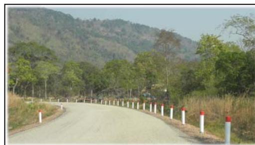
Fig.38, 39: (before 2017 and after 2008) winding access road midway to the temple on the top. On the left road in construction 2008, on the right road after rehabilitation, it is in reinforced concrete in 2009, (by Author).
