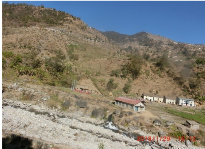
Fig. 1.8 Micro hydro power plant (Potmara, Kalikot, Nepal)
