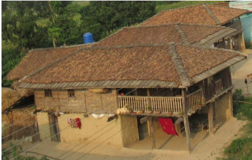
Figure 3.6 A sample of bamboo walls and tile roof.
